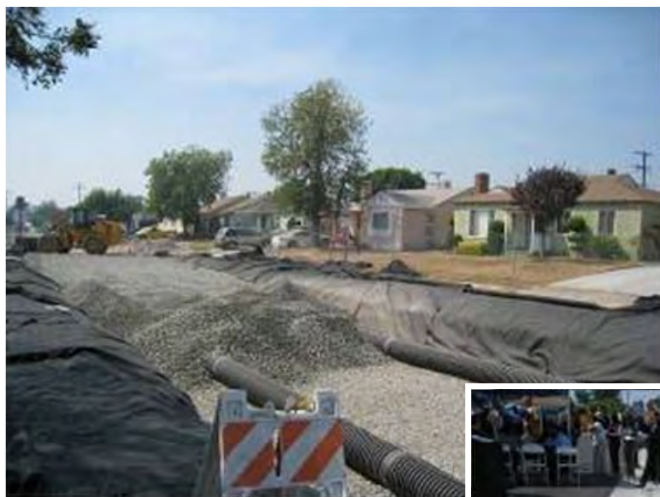
Infiltration galleries under street
