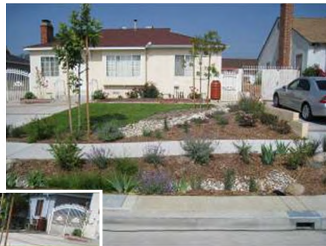
Rain Barrels, Rain garden bioswales & porous pavement
