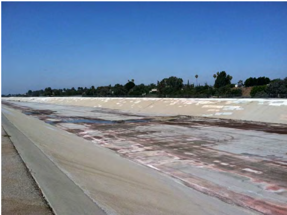
Rio Hondo Channel (a concrete-lined hard-bottom trapezoidal channel)
